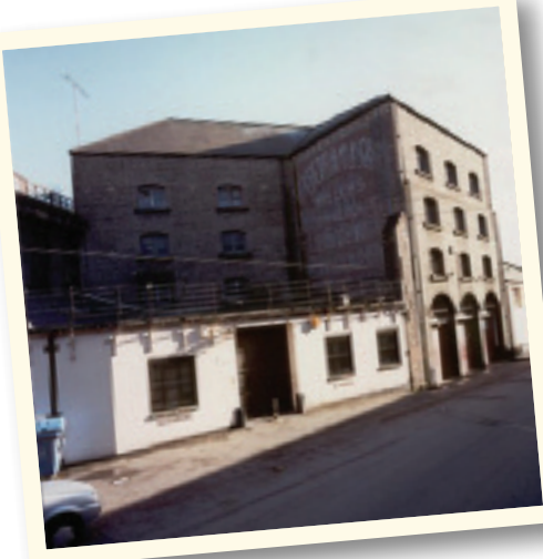
The Seven Stories site before work began.
